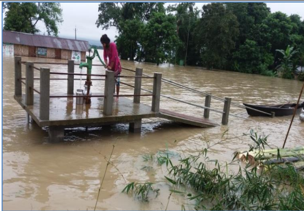
The raised hand pump in Nepali Pathar under Muktiar GP
